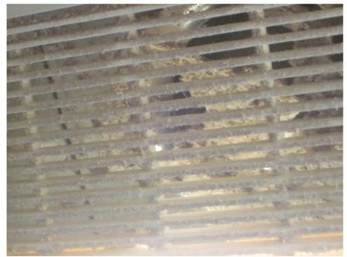
**Attention Needed** - There is an exhaust fan installed in this bathroom, but it does not appear to be removing air at a satisfactory rate. Cleaning or repair is indicated.
