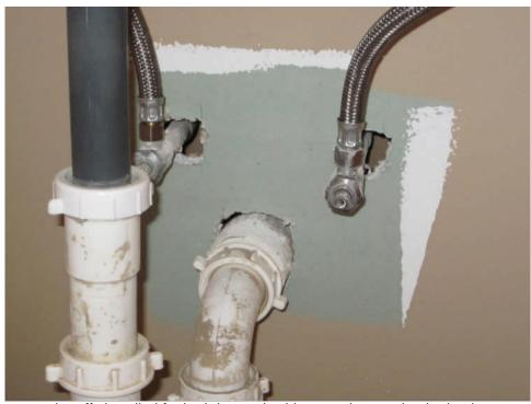
There are no shutoffs installed for both hot and cold water pipes under the basin.
