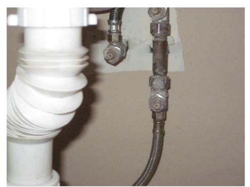
There are no individual shutoffs installed for the supply lines under the sink in the basement kitchen.
