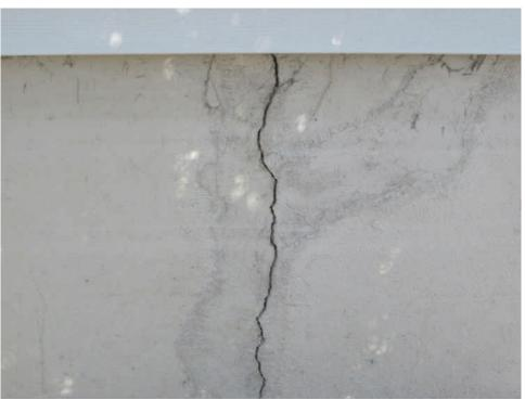
Vertical cracks were noted in the left side exterior wall. Repairs have been made in the past. This home has been flooded in the past.
