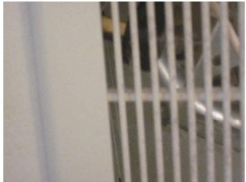
The electric to the fan is disconnected- The ventilation fan vents into the attic space. This introduces moisture into the attic that must be removed from the attic. It would be better to vent the bathroom to the outside rather than the attic.
