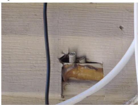
**Attention Needed** - The exterior siding material or finish is in a condition that requires minor repair to prevent further deterioration.
