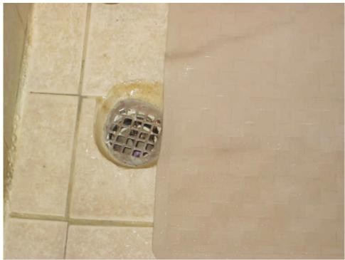
The drain is not installed properly. You can cut yourself or trip.
