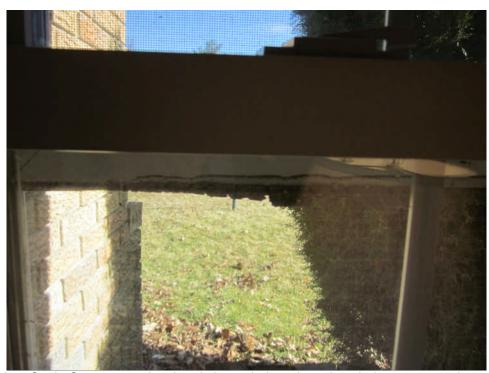
Insulation Seal - One or more insulated glass windows have lost their vacuum seal. As a result of losing this seal, condensation between the two panes creates a clouded or streaked appearance. The window still performs the task of keeping the weather out, but it has lost much efficiency.
