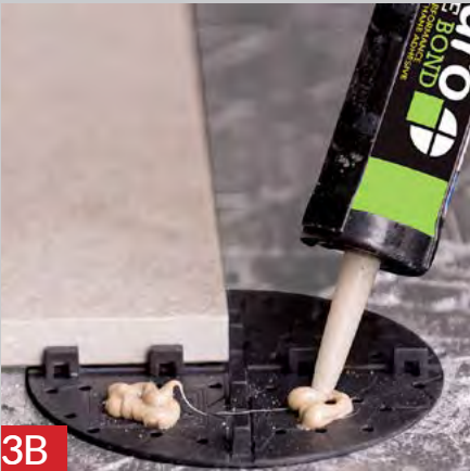
Installation of Everblue Tile and Gator Spacer
