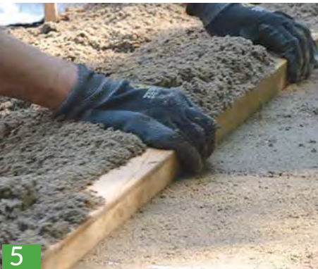
Levelling the Bedding Sand
