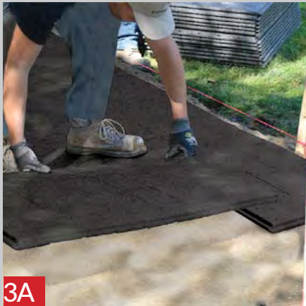
Installation of the Gator Base
