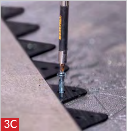
Installation of Gator Edge and Screws
