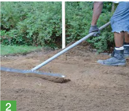
Levelling of the base
