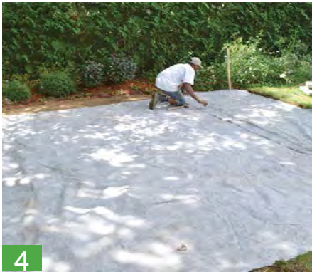
Addition of geo-fabric
