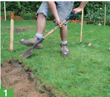
Excavation of the new area
