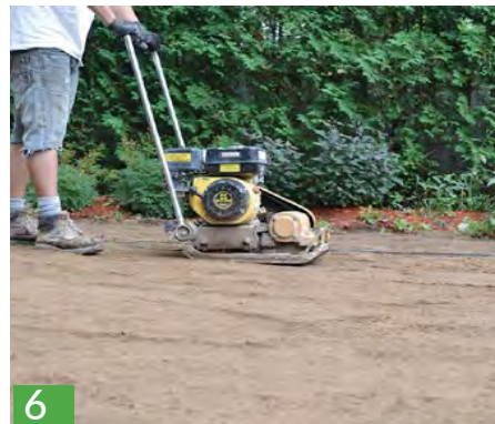
Compacting the Bedding Sand
