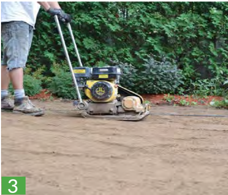
Compacting the Base
