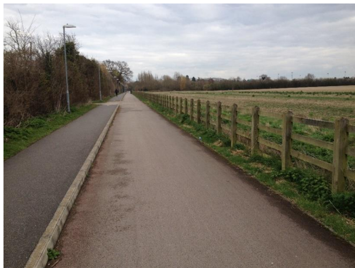
Cycle track in Cambridge, with clearly defined space for cycling and walking ( Location )
