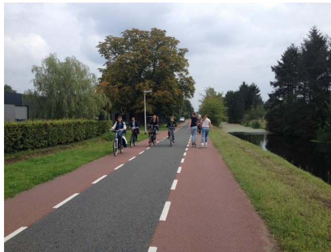
Former main road outside Assen, The Netherlands. Part of a main cycle route with access maintained for motor vehicles ( Location )
