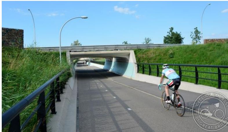
Cycling and Walking underpass in Zwolle, The Netherlands (Picture credit) (Location)
