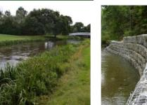
Pre planted coir rolls in combination with a gabion basket terrace will protect the riverbank from erosion in this location whilst the pre planted rolls and seeded gabions will soften the engineered appearance and provide a viewing platform towards Allington Castle.
