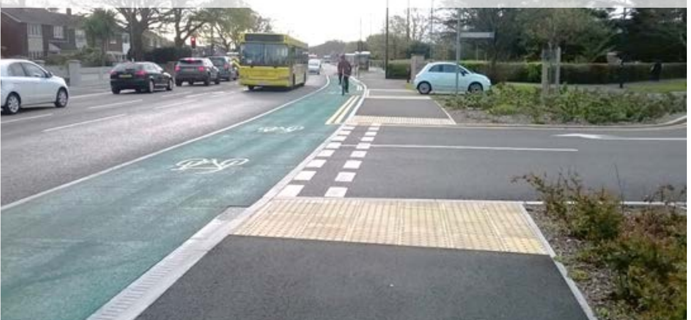
Figure 10.17: No setback crossing with design priority,– Bournemouth
