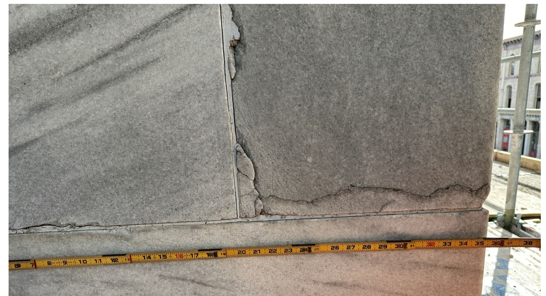
Marble damage at joints
