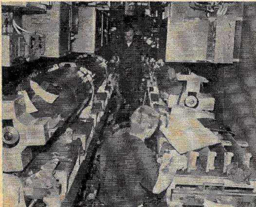
TORPEDO CREW readies "fish" for mock attack on enemy. High-pressure water ram pushes torpedo from tube, catapulting it out for run on target
