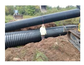
Pictured above is Bob Rynders replacing a rusty 5' steel culvert with three 3' polyurethane tubes.
