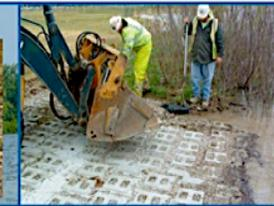
Armor—flex holds soil and provides a hard, porous surface which can support grasses and foot traffic.
