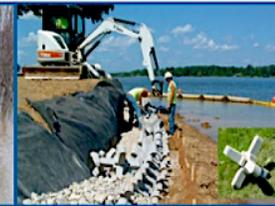
A-jacks stabilizes severe bank erosion and allows interspersed plant growth for added protection.
