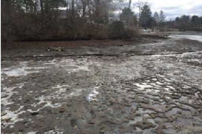
This picture was taken in Cove C – south shore in January 2018. Note the silt build-up and the shadow where the embankment has significant erosion issues.
