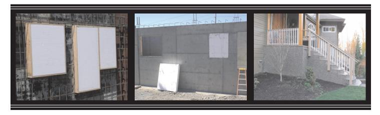
**Form Follows Function...** The EPS Block-Outs were used to help frame the window and door penetrations of this poured in place wall. After the forms were removed, the EPS Block-Out was also removed and used again as a light weight fill, to reduce the mass of the stairs and decks on the project. The contractor saved on material costs, labor costs and accelerated the construction time.
