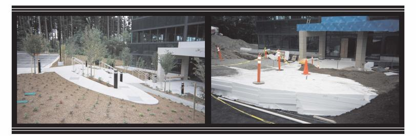
Using EPS Block-Outs for concrete decks, ramps and stairs, not only reduces the amount of concrete, but lighter concrete mass means a smaller footing can be used, with less weight against a building's foundation.
