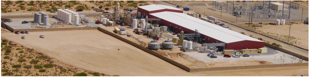
Figure 2. Photo of the Full Recovery Desalination ® plant in El Paso, Texas. (Courtesy of EWM 2019)
