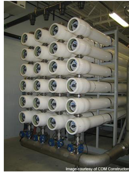
Figure 2: Sand City Desalination Plant compressed reverse osmosis skid. (Desal-14-06)
