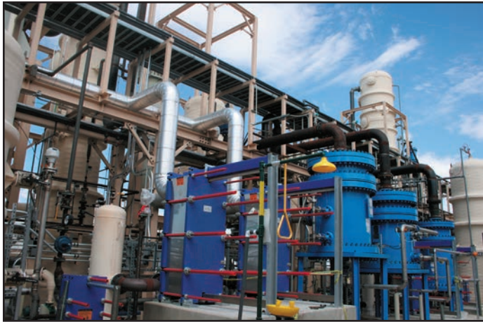
Enviro Water Minerals' concentration system processes the diluted chemicals manufactured in the plant. They are then concentrated to commercial strengths.
