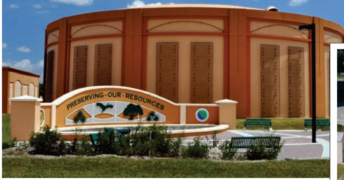
Tanks with Architectural Treatment
