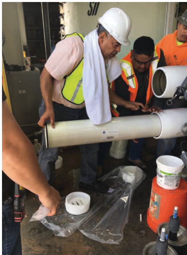
Left: Acid/caustic heat exchangers and evaporator installation Right: Installation of demineralization membranes Photos by Bill Norris, NorrisLeal, taken in March 2017.
