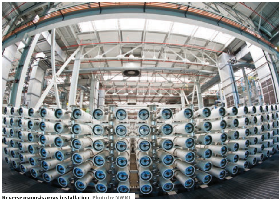
Reverse osmosis array installation. Photo by NWRI
