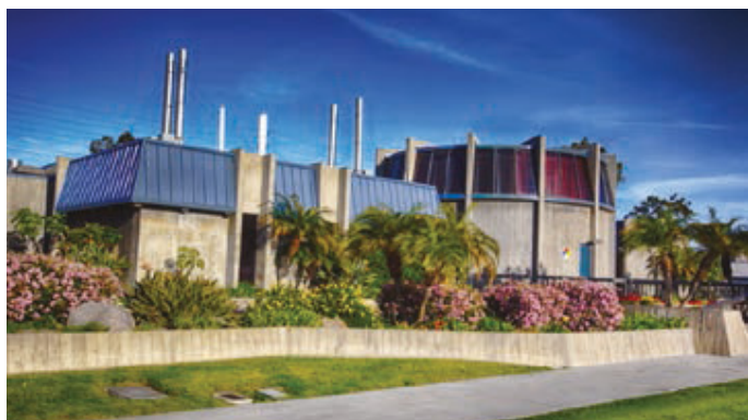
In Los Angeles, California, the Terminal Island Water Reclamation Plant's expanded Advanced Water Purification Facility (AWPF), now under construction, will be the first greenfield AOP design using UV light with chlorine for indirect potable reuse. Photo by Xylem
