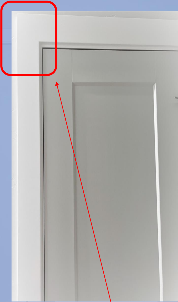
"Flush Mount Style" Door Trim (45-degree cuts) (MDF Wood) Included in Price
