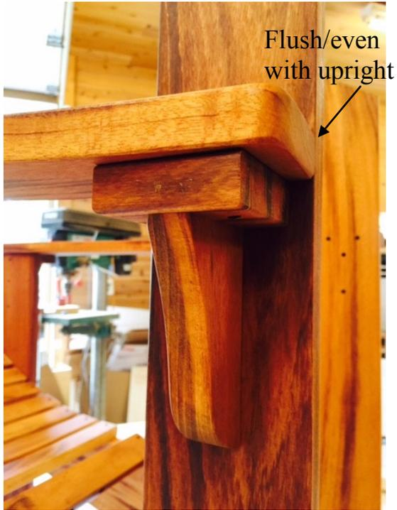
**8-**Attach the front of the arm to the front arm support by positioning it so there is approx 1/4" overhang to inside of the front leg . Pre-drill and install 3- 1 1/2" thru top plate of arm support and into the arm.
