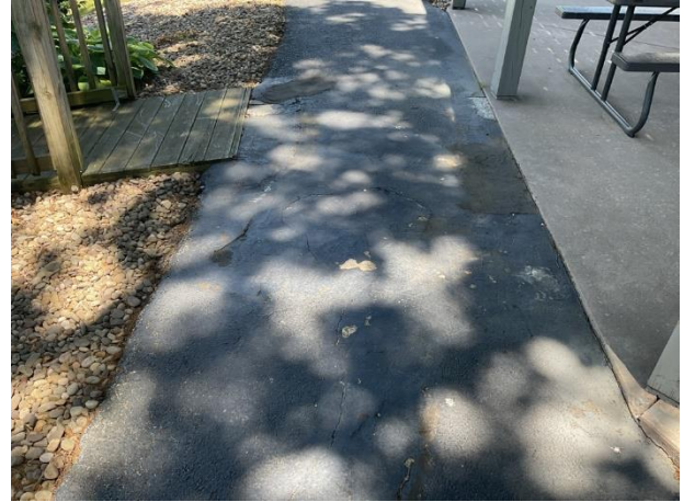
Previous settlement repairs
