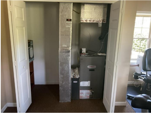
Split system air handling unit
