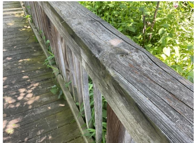
Wood deteriorating
