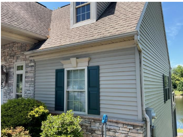
Aluminum gutters and downspouts
