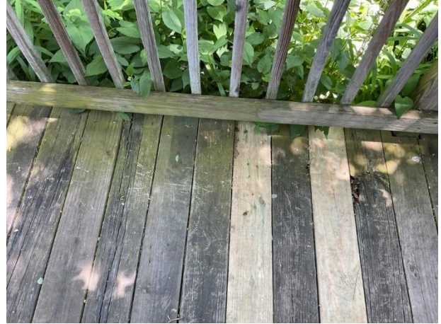
Previous repairs, wood rot and organic growth
