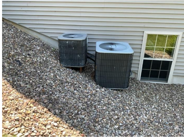
Split system condensing units
