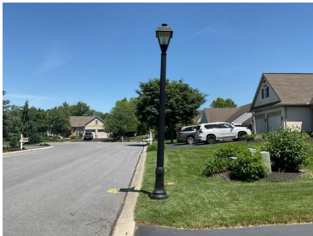
Light pole and fixture - note leaning pole
