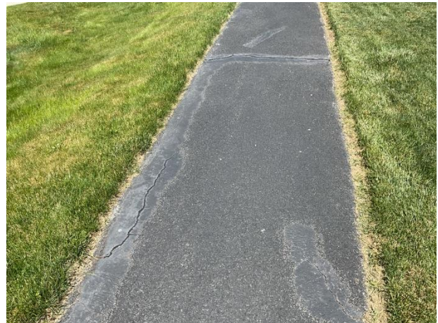
Walking path cracks
