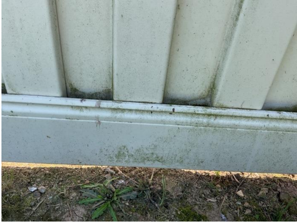
Organic growth and finish deterioration
