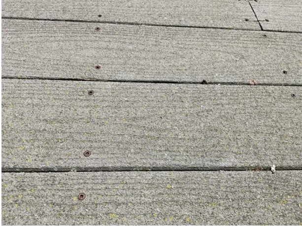
Composite decking surface deterioration
