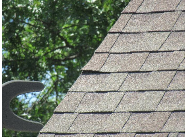
Isolated shingle lift
