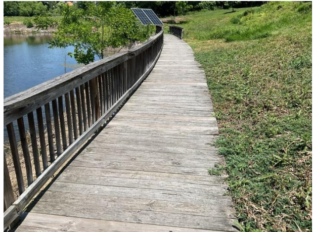
Wood deterioration
