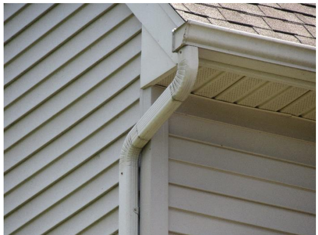
Aluminum gutter and downspout
