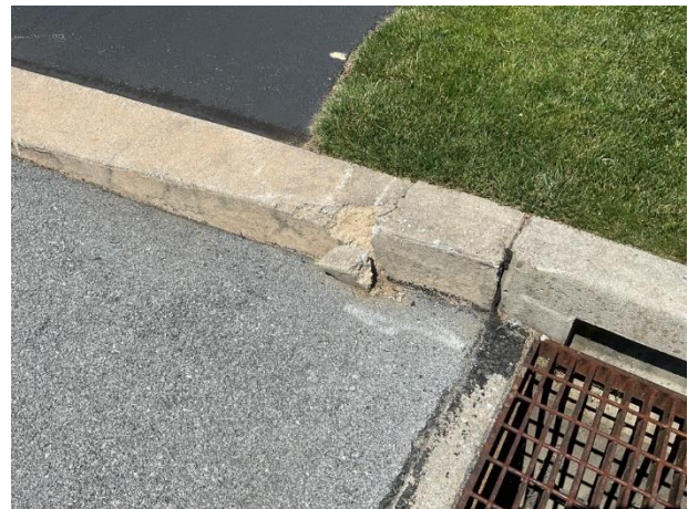
Concrete spall
