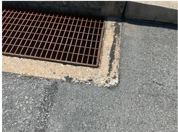
Concrete spalls
