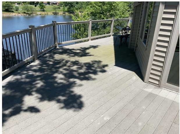
Composite decking - Note surface deterioration and organic growth
