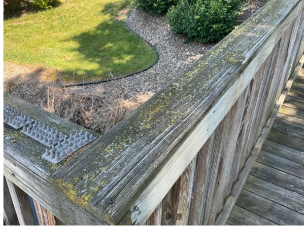
Organic growth and wood deterioration
