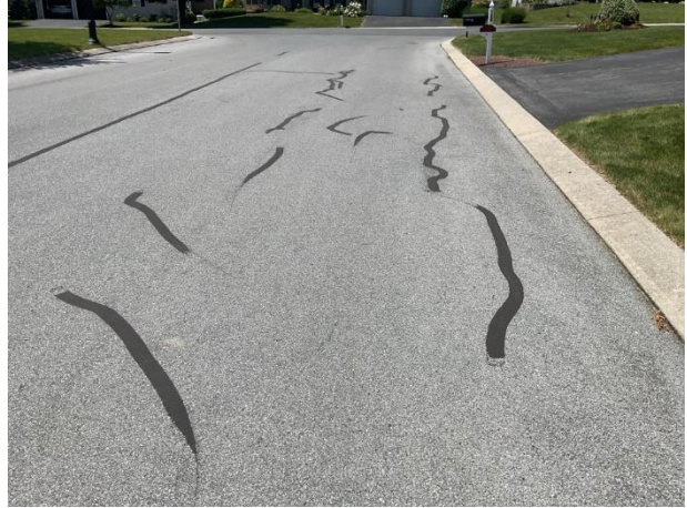
Previously repaired cracks – Lantern Drive
