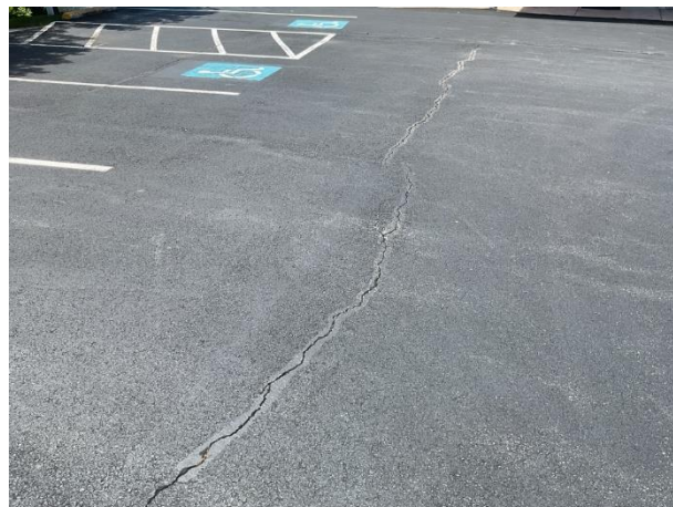
Pavement cracks – Parking area
