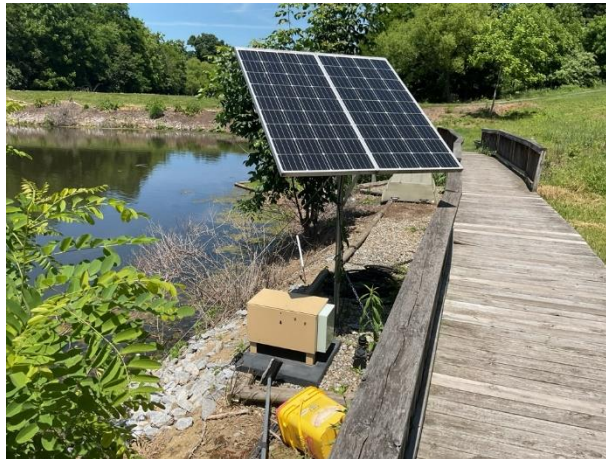
Aerator pump and solar panels
