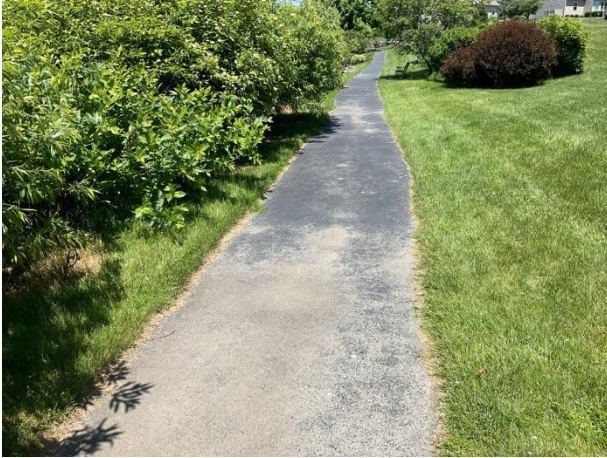
Asphalt pavement walking path - Note seal coat deterioration
