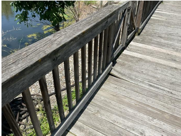
Wood deterioration
