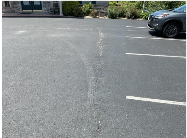
Pavement cracks – Parking area
