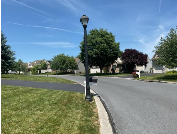
Light pole and fixture - Note leaning pole
