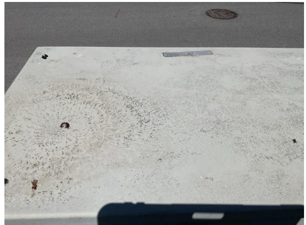
Mailbox station finish deterioration
