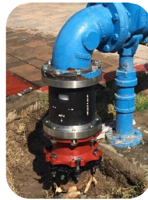
SMART VALVE™ Installation
