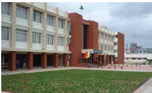
Development Work at IIEBM, Hinjewadi, Pune, Maharashtra
