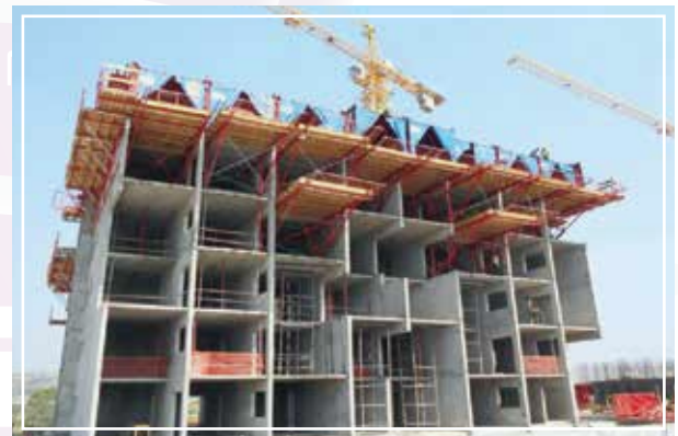
TUNNEL FORMWORK
