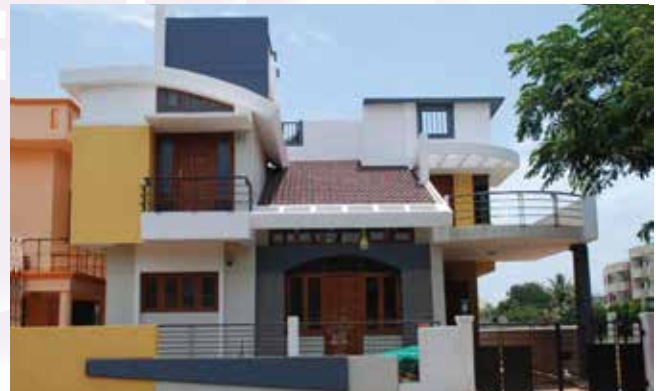
Residential Project for Wahile, Chakan, Maharashtra
