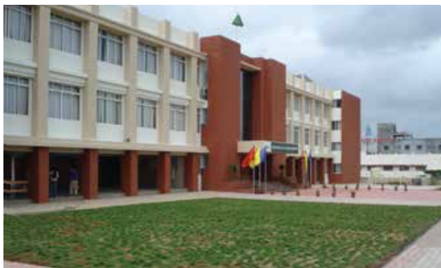
Development Work at IIEBM, Hinjewadi, Pune, Maharashtra
