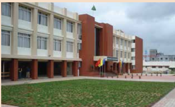
Development Work at IIEBM, Hinjewadi, Pune, Maharashtra
