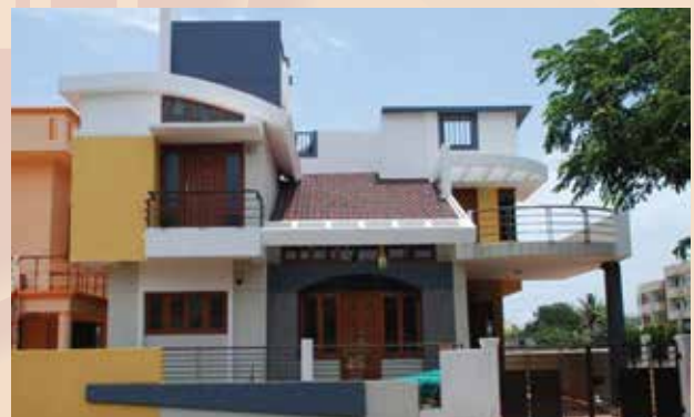
Residential Project for Wahile, Chakan, Maharashtra
