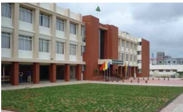
Development Work at IIEBM, Hinjewadi, Pune, Maharashtra
