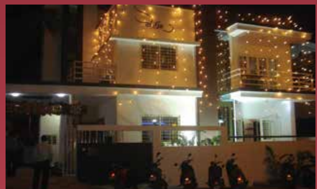
Bungalow Project at Nigadi Pradhikaran, Pune, Maharashtra
