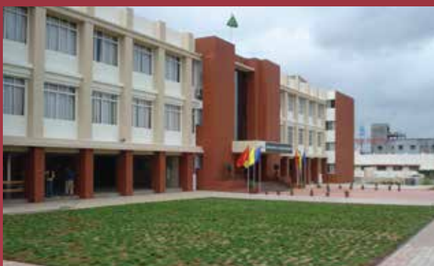
Development Work at IIEBM, Hinjewadi, Pune, Maharashtra
