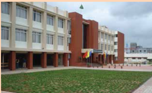
Development Work at IIEBM, Hinjewadi, Pune, Maharashtra
