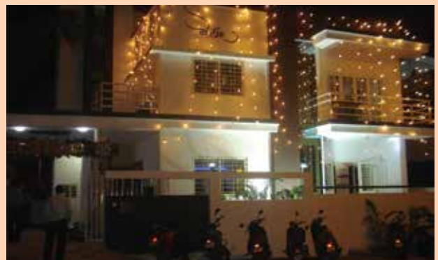
Bungalow Project at Nigadi Pradhikaran, Pune, Maharashtra
