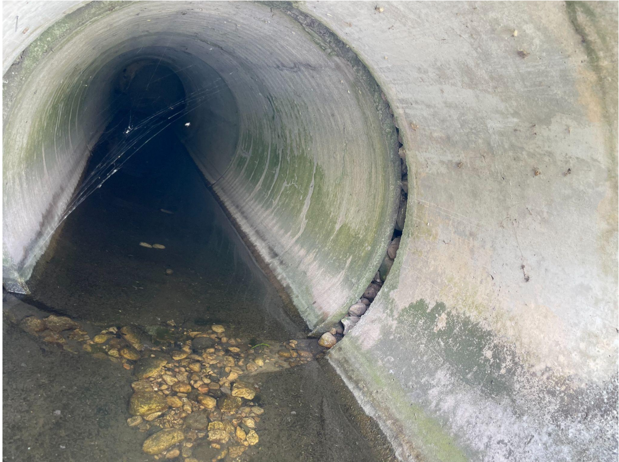
Image 8: Lot J detached flared end section. Will cause significant erosion damage if not corrected.
