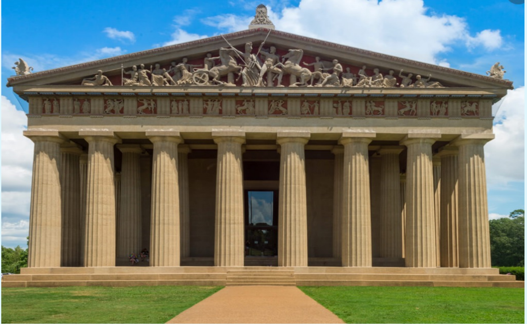
The Parthenon, Nashville, TN Built in 1987 for the Tennessee Centenary Exposition
