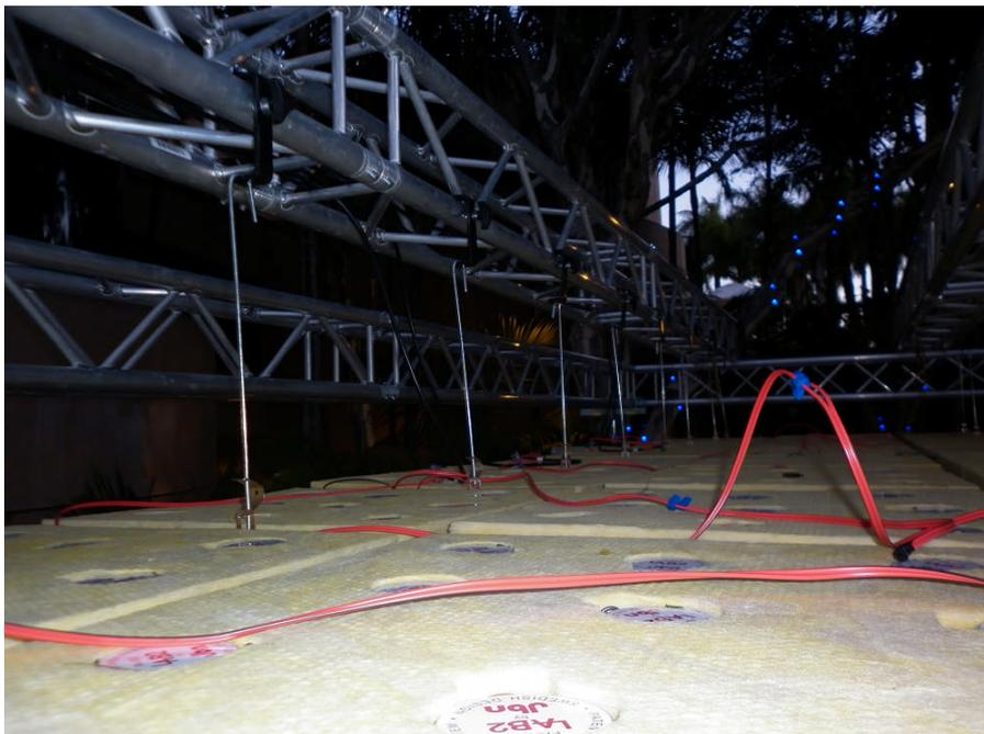
**Figure 2 – Sound Ceiling panel from above**
