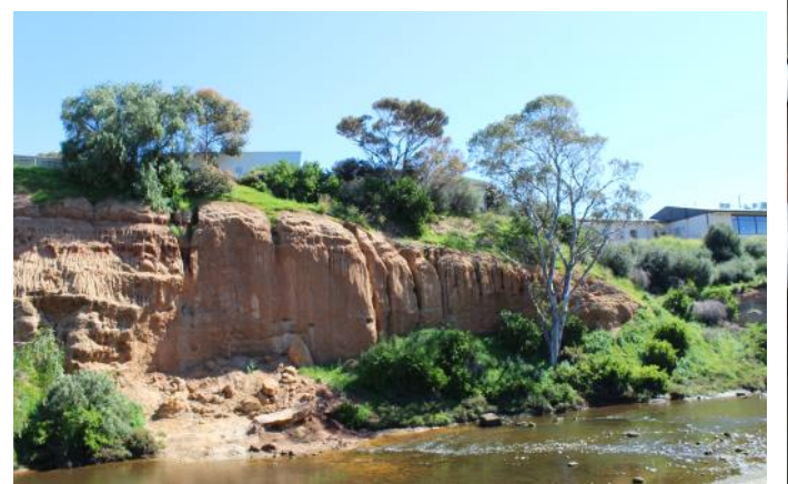
A few metres further on is an area where the cliff face is suffering from erosion and collapsing showing the dangers of building too close to the edge!
