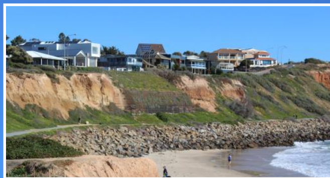
The cliff defences from a distance seem to be successful by 2021 in encouraging vegetation and stabilising the cliff...
