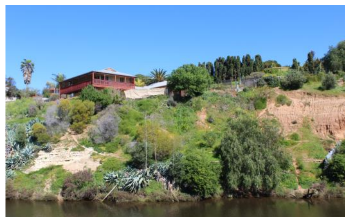
Homes built close to the edge of the cliff. The white area is the limestone of the Blanche Point Formation about 55 million years old. The red area next is of much younger less than 10,000 year old clays.
