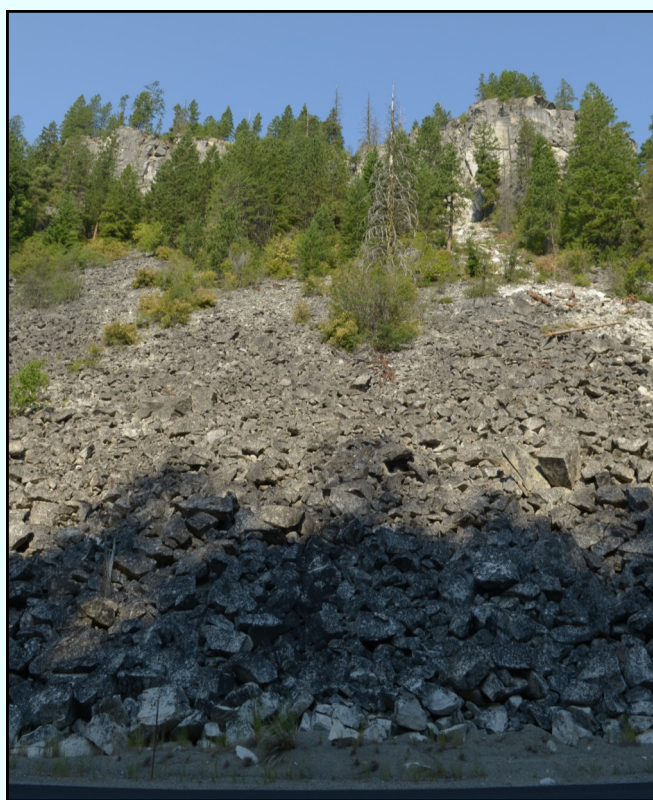
FIGURE 2. Talus Slope near Omak, Washington Large, angular blocks of basalt have tumbled a short distance down a steep slope, forming a cone of debris. Photo by Susan Celestian
