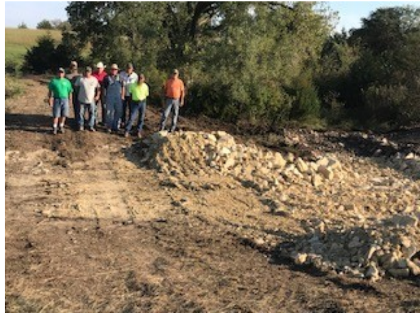
Completed repair. Rock here and on culvert crossings provided by Bayer Construction Company.
