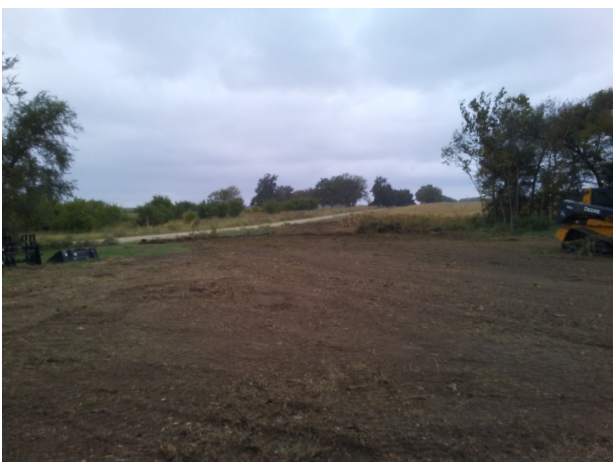
Cleaned up headquarters and roadway to allow for power line installation.
