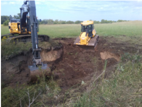
Starting work on emergency spillway repair - as you can see there is quite a wash out that was only a couple feet from taking the pond out.
