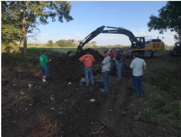
Working on the narrow crossing a combine can't get through with the header on.
