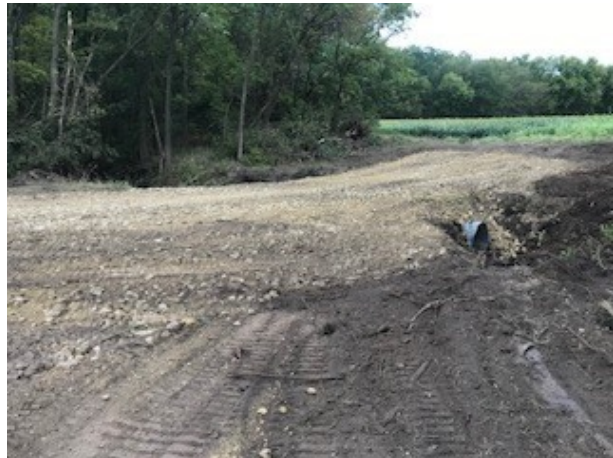
Completed with culvert extension and room to clear the header.
