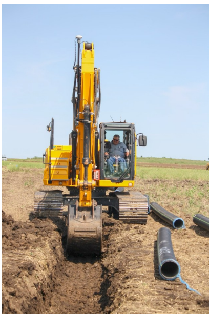
Joe trenching for pipe at the SAVE Farm.
