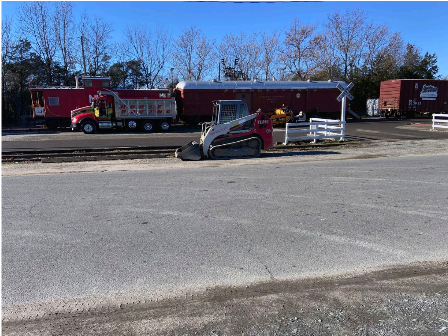
House Paving Co. installing new surface on parking lot 12/12/2023
