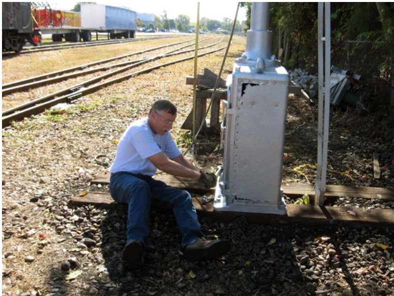
Flash back to Oct. 10,2007. #1 Don K. bolting signal in place
