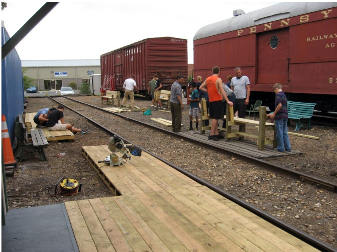
9/22/2025 Boy Scouts build platforms and benches at Deep Run Station.
