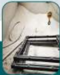
4 Sand Blasting Treatment
