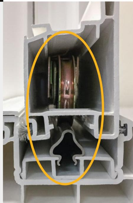
Door rollers glide over a durable, one-piece stainless steel track with effortless operation for a lifetime.
