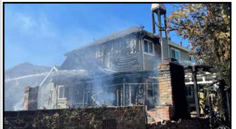
Just before noon on May 24th firefighters from Santa Clara County Fire Dept. responded to a structure fire on the 300 block of Harrison Ave. The fire caused significant damage to the detached structure at the rear of the property as well as causing damage to the house behind the property that was located on Central Ave. A small fire also started on a wood shake roof several doors away from the falling embers but was quickly extinguished. Photo: Courtesy SCCFD.
