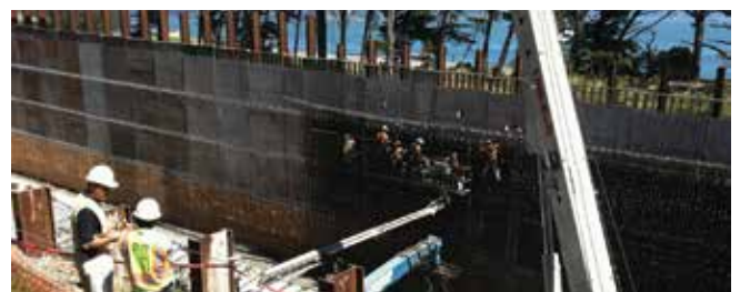
Blind Side Waterproofing
