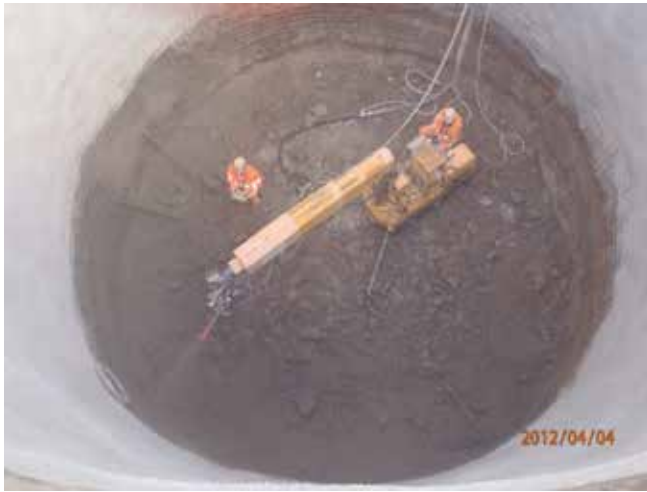
Fig.4: Normet spraying manipulator in action
