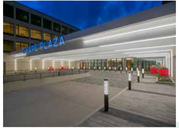
O'Hare Plaza West Drive and Executive Garage Restoration | Chicago, IL
