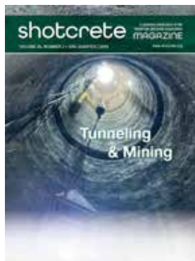
Ventilation shaft from the excavation pit of a long road tunnel in the southern German Alps with an 18 ft (5.5 m) diameter and 279 ft (85 m) depth. Noted in "The Application of Shotcrete in Shafts", Pg. 10.
