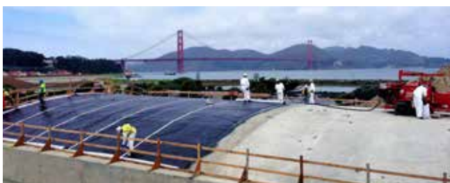
Positive Side Waterproofing
