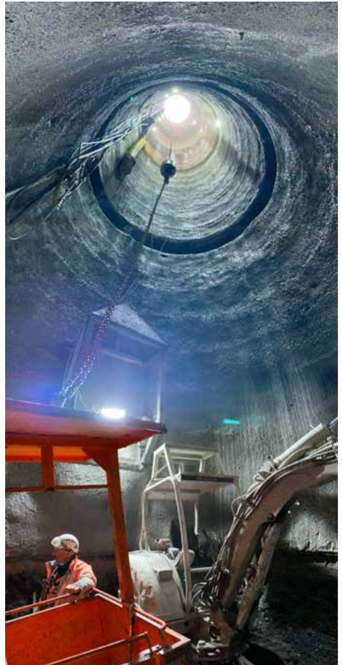
Fig.1: ventilation shaft from the excavation pit
