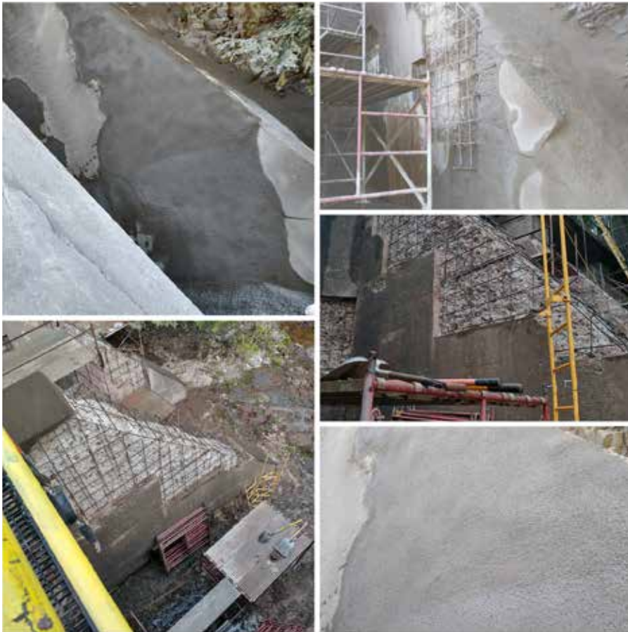
Left & Above: During the restoration of a dam Near Lake Superior, dry-mix shotcrete was employed based on logistical considerations.
