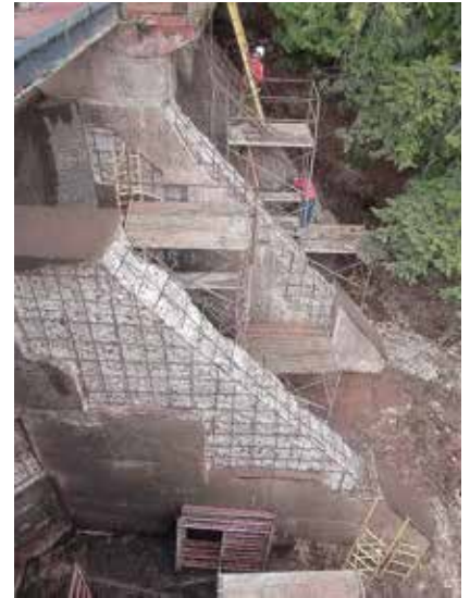
Left & Above: During the restoration of a dam Near Lake Superior, dry-mix shotcrete was employed based on logistical considerations.
