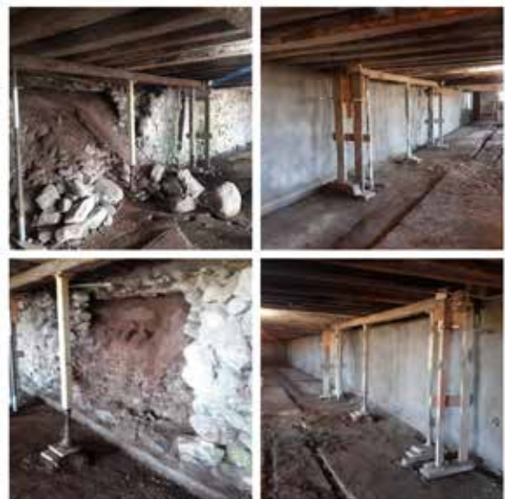
Left & Below: Stone foundation restoration using Wet + Dry Shotcrete
