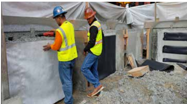
Fig. 2 Installation of the outer fleece reinforced HDPE sheet
