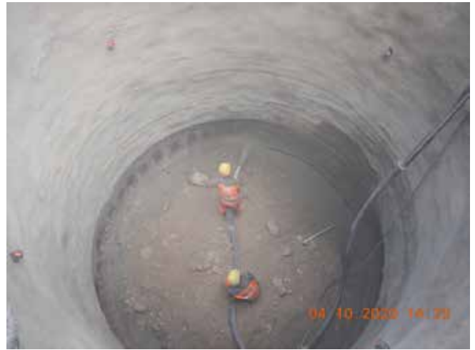
Fig.3: Shotcrete application inside the shaft
