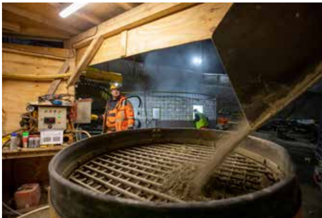
Fig.2: Feeding the Alivia-Pump with shotcrete
