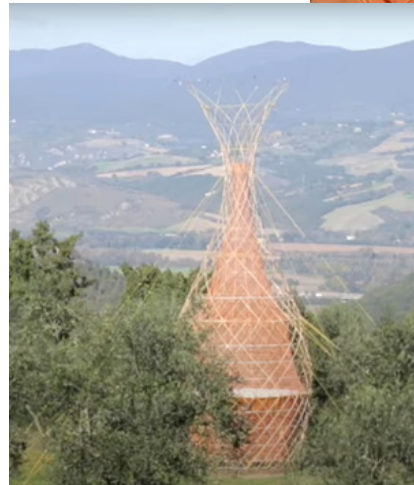
Warka Water towers harvest drinkable water from the air
