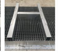
8. The claws should be located diagonally opposite, end-to-end to spread any applied load along the length of the beam. It is now safe to remove the GRP within the area created by the beams.
