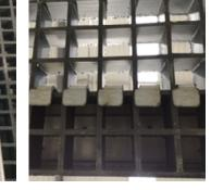
7. Pull the claw in over the top of the beam. Fix in place using the tek screws provided. A minimum of 2 claws per beam should be used.
