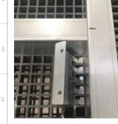
5. Locate the claw next to the 6. Where possible, push the claw cross beam or at the centre of a towards the perpendicular bars support beam, drop it through so that it increases the support the grating and pull it towards the to the GRP panel. beam.
