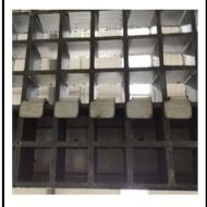
6. Where possible push the claw towards the perpendicular bars so that it increases the support to the GRP panel.
