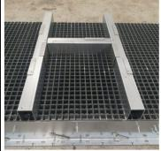
8. The claws should be located diagonally opposite, end to end to spread any applied load along the length of the beam. It is now safe to remove the GRP within the area created by the beams.
