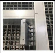
5. Locate the claw next to the cross beam or at the centre of a support beam, drop it through the grating and pull it towards the beam.
