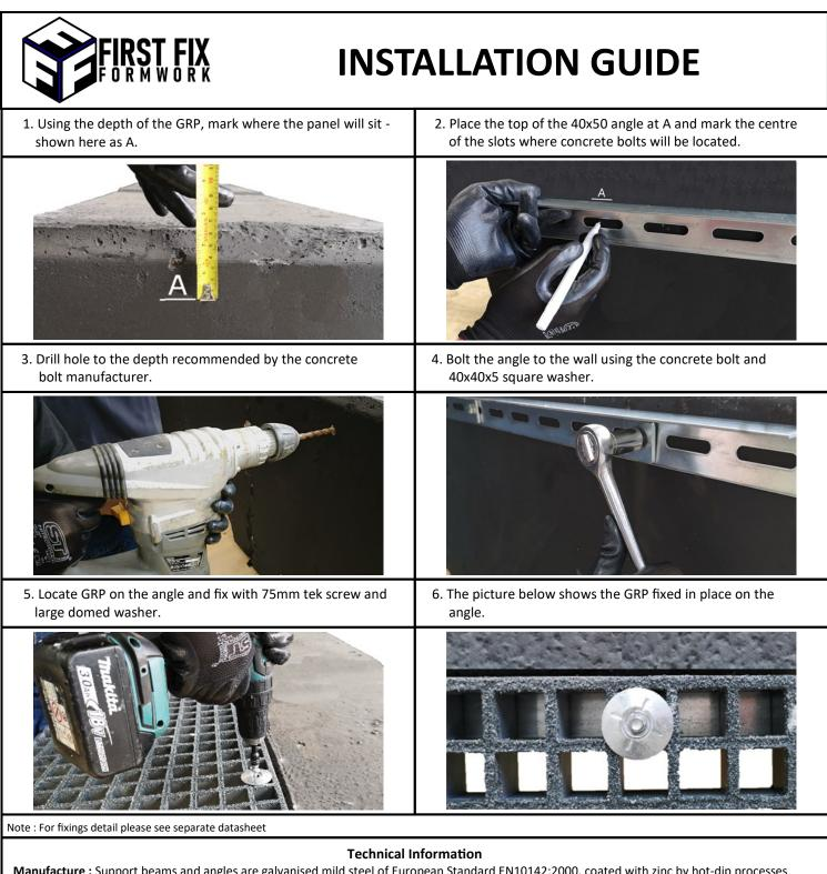
**Manufacture :** Support beams and angles are galvanised mild steel of European Standard EN10142:2000, coated with zinc by hot-dip processes (Galvatite Z), including iron-zinc alloy (Galvatite ZF). The hot-dip coatings may contain up to 0.002% lead or up to 0.12% antimony. Fibreglass grating is made from fibrous glass, polyester resin, catalyst (peroxyester), styrene, aluminium oxide, pigments. Ingredients are chemically cured and bonded together.
