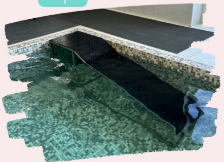
The new pool ramp
