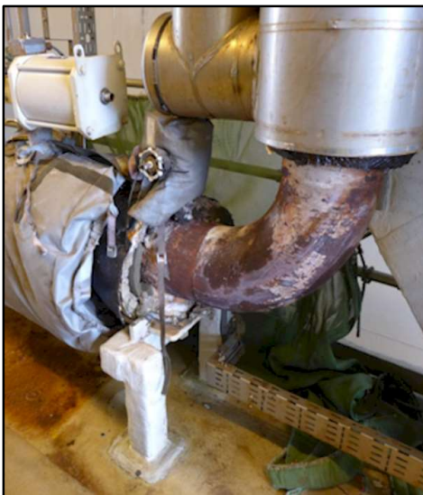
Corrosion Under Insulation (CUI) can be prevented by using ThermaCoat-400
