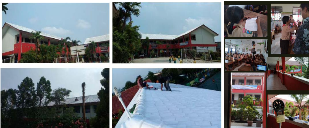
Fig 4. Cool Roofs Application and physiological test at Elementary School
