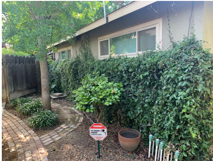
North side of structure
