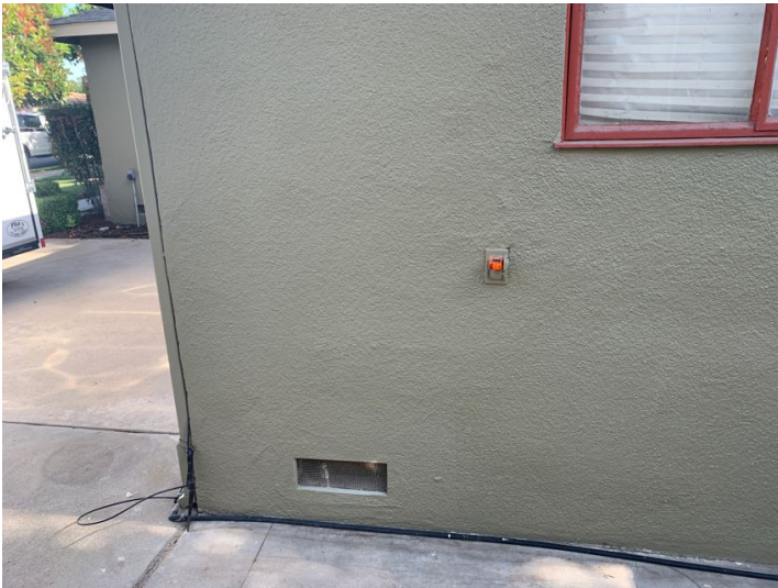
South side of structure
