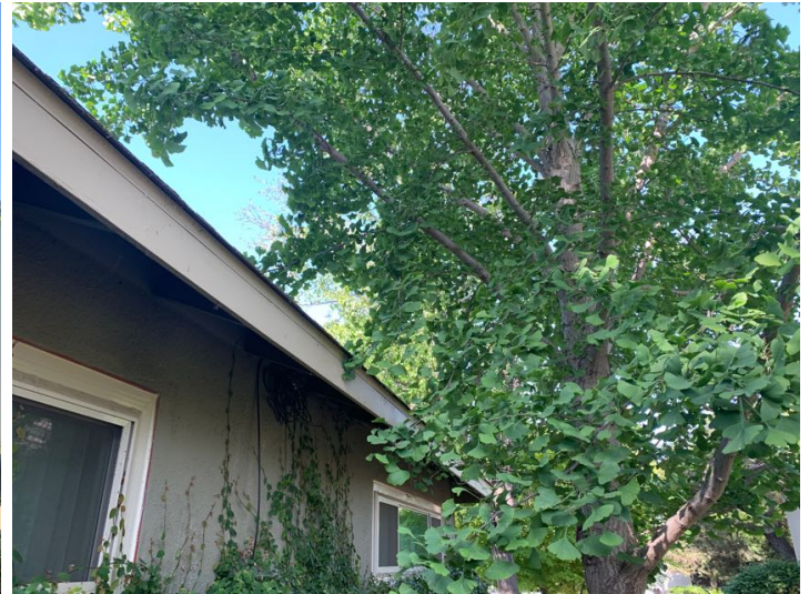
Northside of structure
