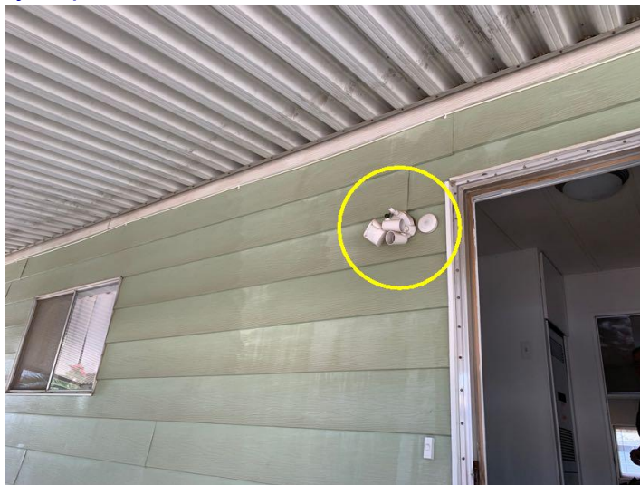
Back entrance door
