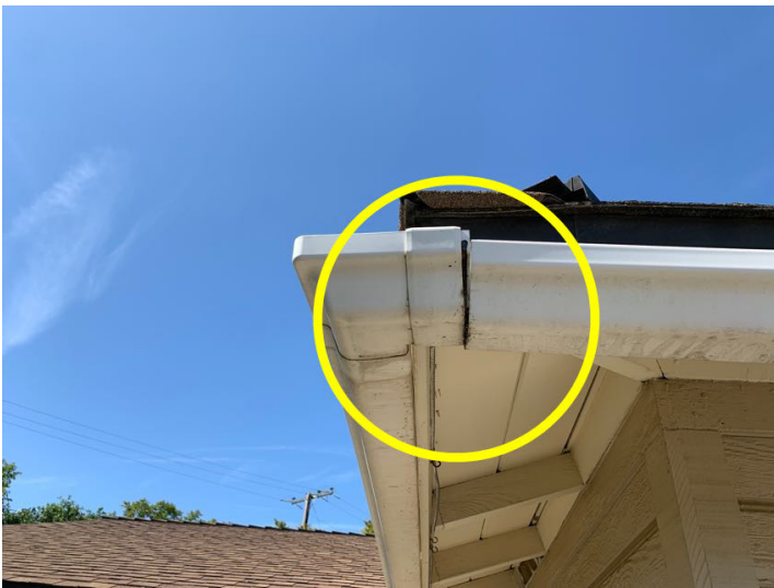
North center of structure
