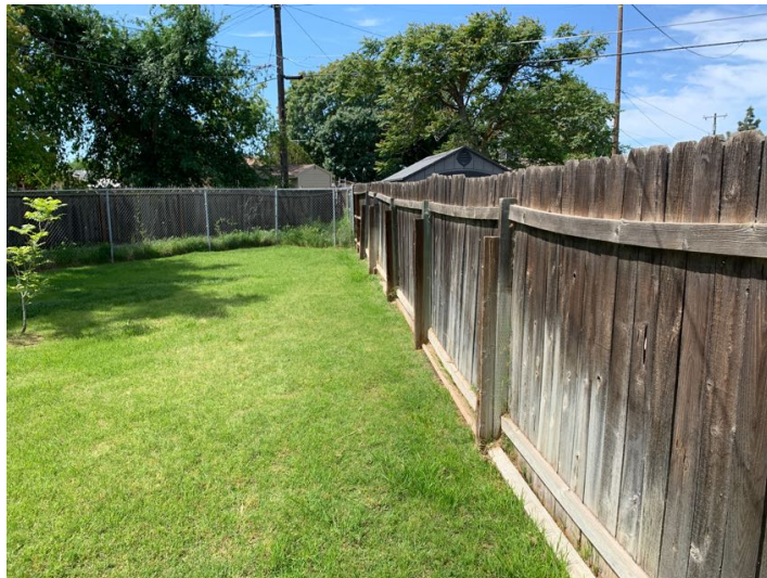
North fence line
