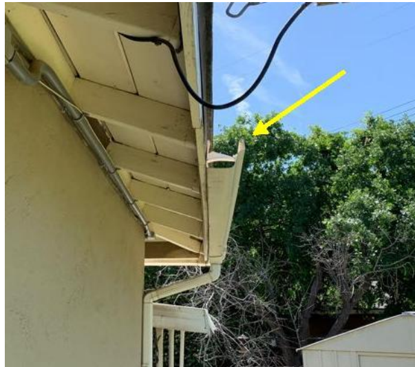
Southside of structure
