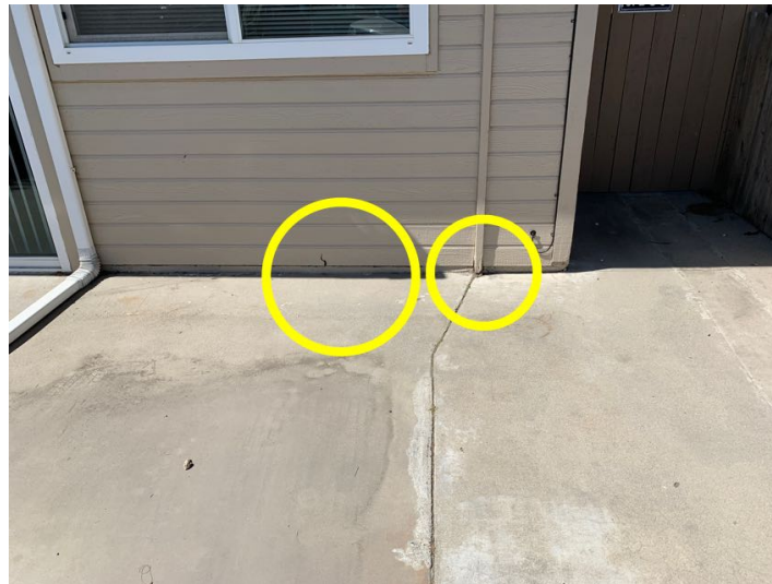
Northside of structure
