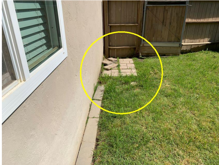
North East corner of structure
